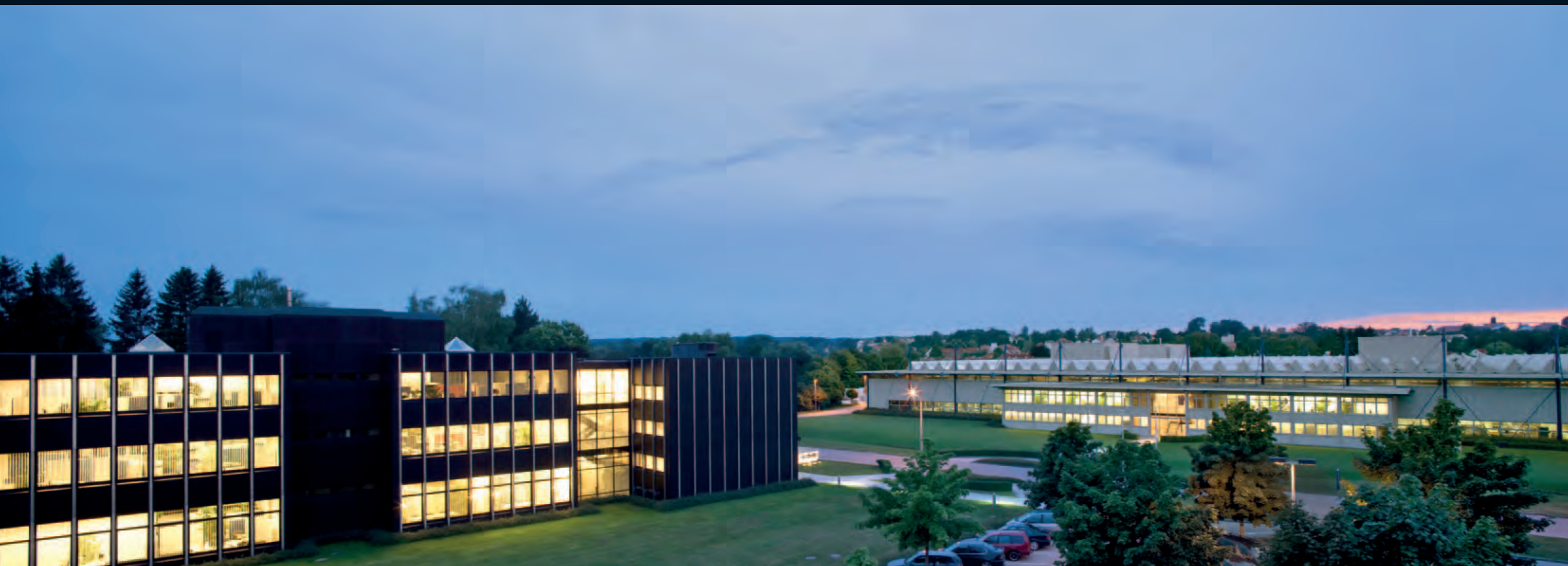
Head Office in Burgau, Germany
